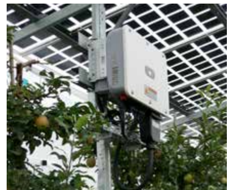
Safe mounting of inverters
