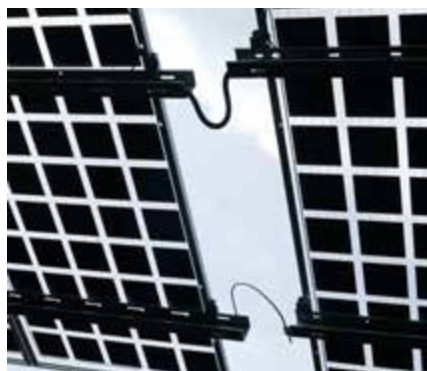
Simple electrical connection of the module tables
