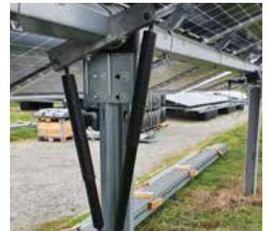
Robust and durable drive on solid foundation according to static calculation
